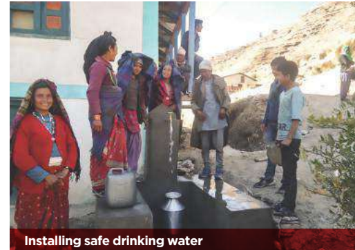
Installing safe drinking water
